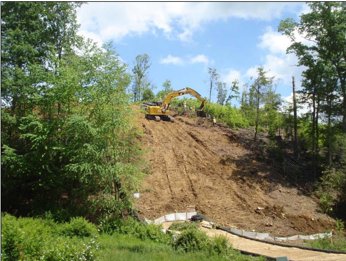
Erosion protection on north side of MVP-mi 246.5 is inadequate, 5/24/18 Bob Peckman
