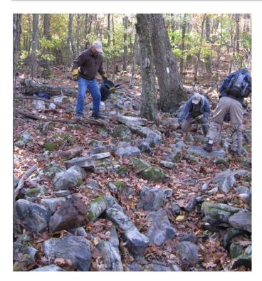
Instead of having to find and move rocks to construct steps, this project was to rearrange the jumble of rocks to provide a better path. Rock bars, leather gloves and sledge hammers aided the hands that hefted, flipped and rearranged the rocks. The effort stoked the internal furnaces, and layers of fleece, pile, flannel and wool were taken off and set aside.
