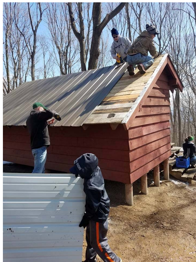
Meanwhile, Jim led a crew working on the water trail. They installed 14 steps on the water trail and
