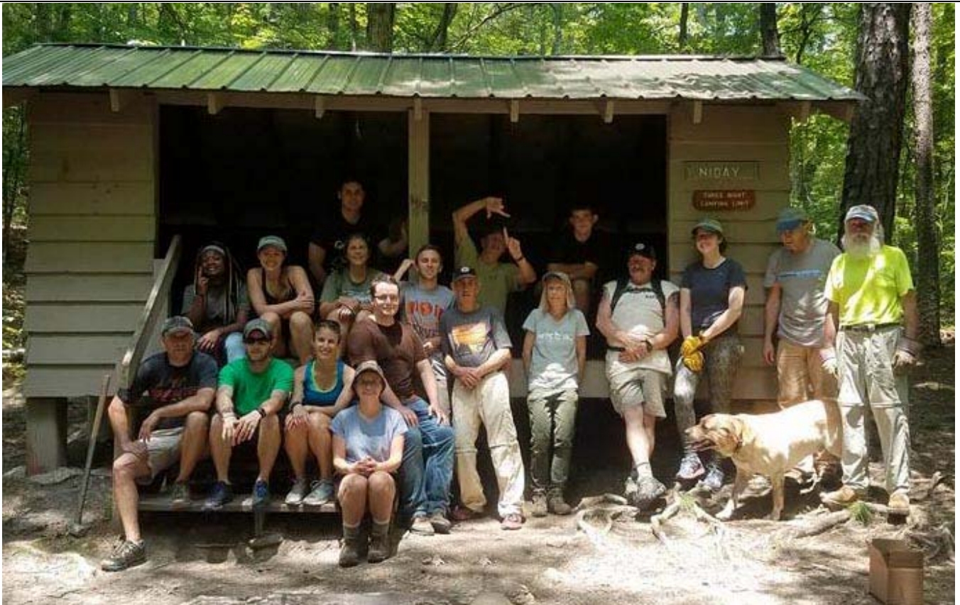
The whole shelter re-roof crew----- Taylor
