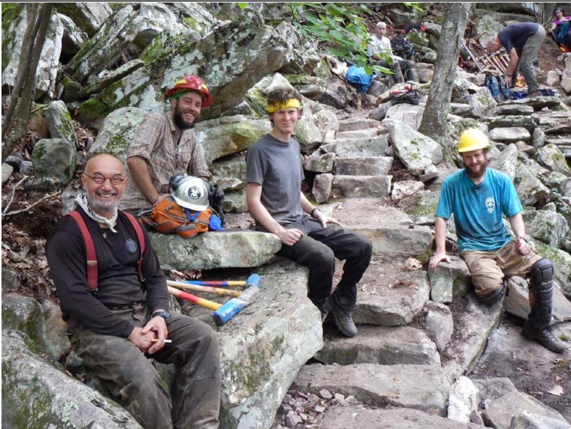
Konnarock began on Sinking Creek relocation in 2016 and will continue through the 2018 season.
