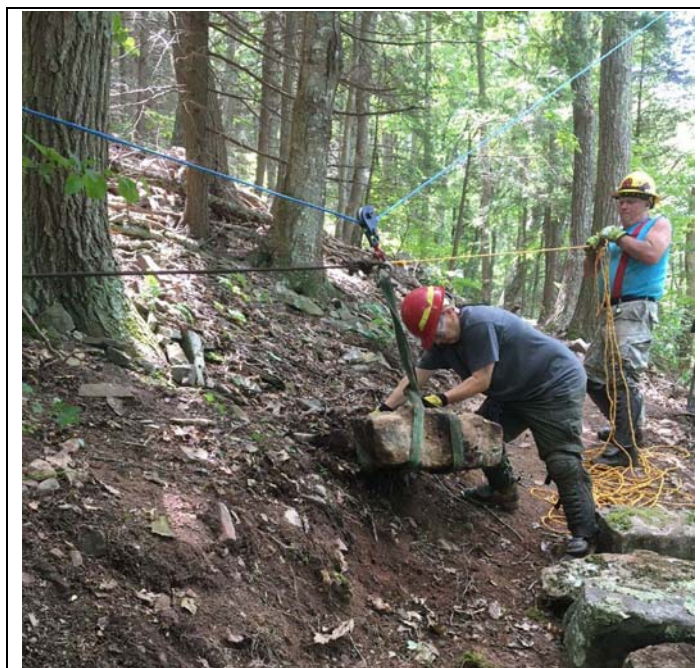
Pulley hangs from blue line, black & yellow lines control it. Webb
